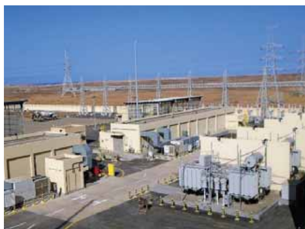
400kV substation
